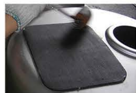
When applying the pad to the sink, a roller is used to flatten or even out the pad.
